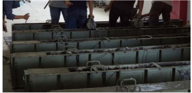
Fig. 3 Casting of Specimens
